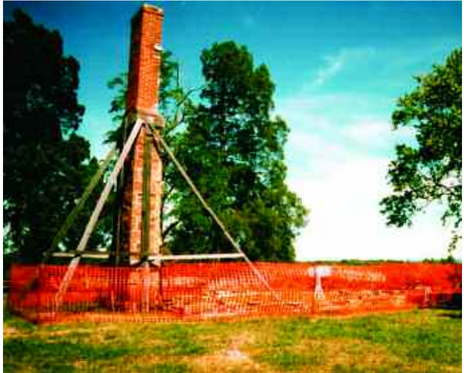
Figure 2: The remaining Robinson House Chimney after the house was dismantled by the NPS following a fire that damaged the structure.
