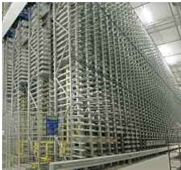
Figure 2. Temporary storage area, ADB Bern, ©ADB Badri Redha.
