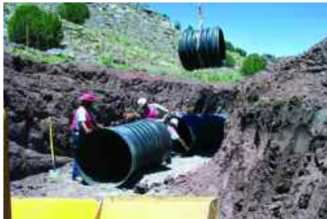
Figure 3: Navajo workers install a segment of pipe for the new irrigation system (Bureau of Reclamation photograph).
