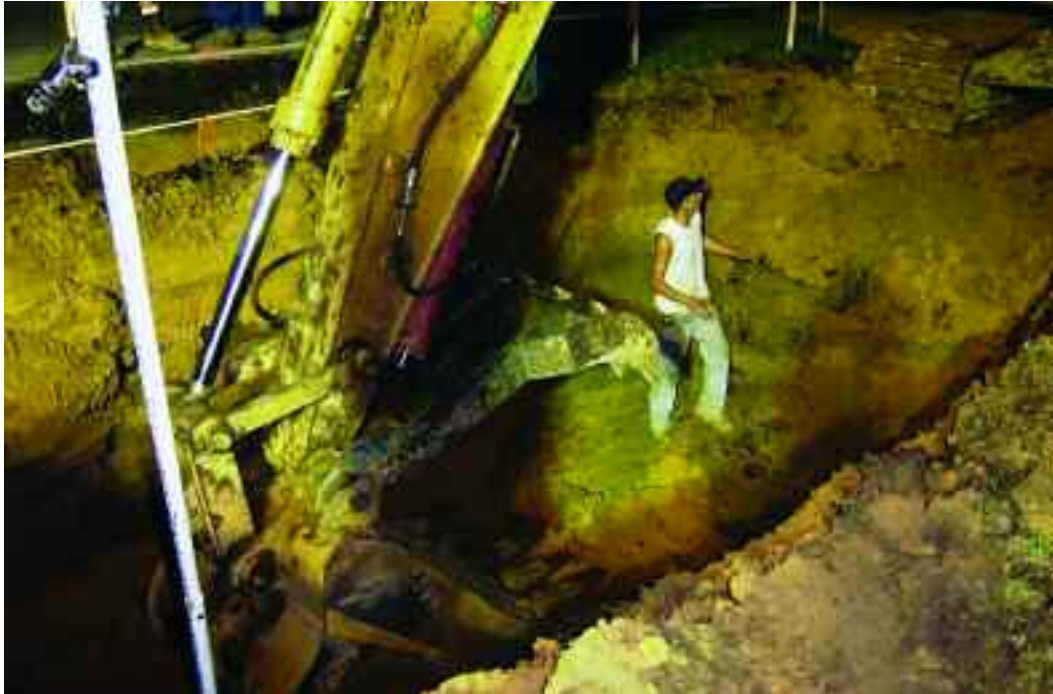
Figure 2: Monitoring of development projects, although often tedious and at odd hours, has yielded important information. In this photo, the hoe is excavating for a sewer along a public road to serve a new office building. The hoe has just uncovered the base of a brick foundation 10 feet below grade, where the man is standing. The profile along the road revealed two or three earlier roads, the first made with tar and chip around 1923, at more than 9 feet below the present surface.
